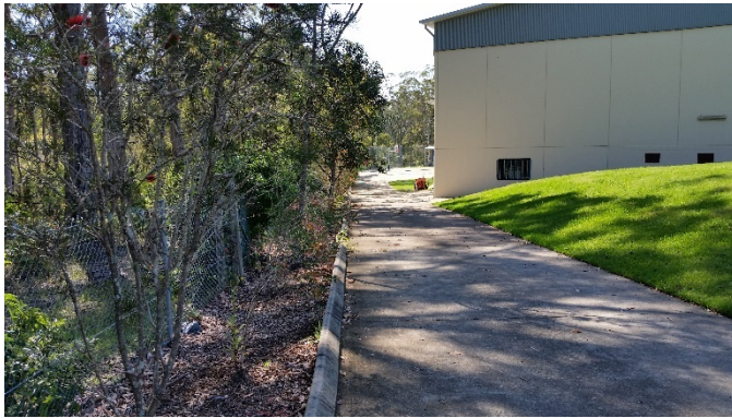
Photo 5 – View to north-east of site along concrete driveway. MPC shown to left of photo
